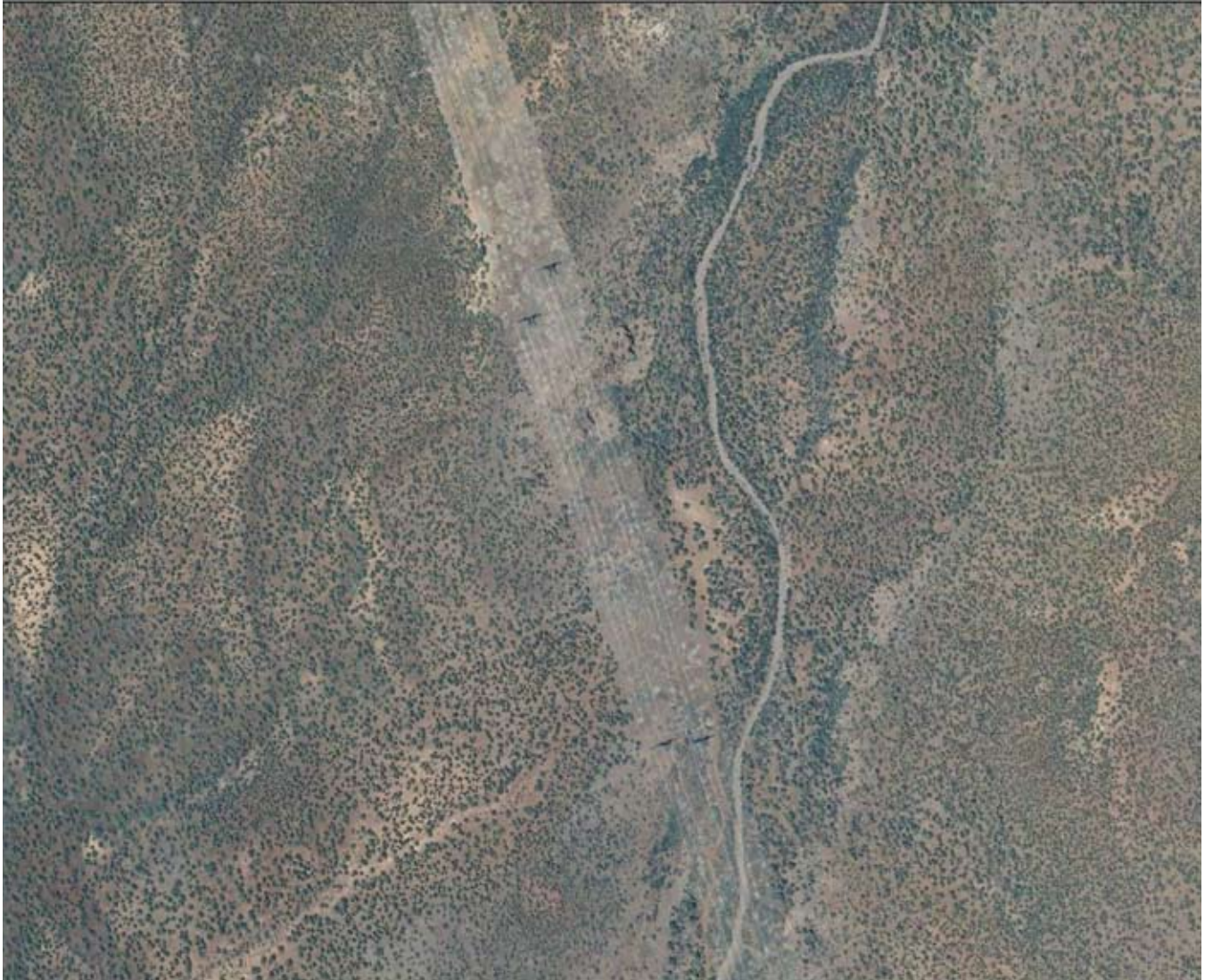
Figure 1. Vegetation maintenance under dual 500-kV transmission line, Prescott National Forest.
